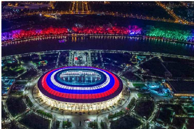
Luzhniki Stadium media roof, Moscow
